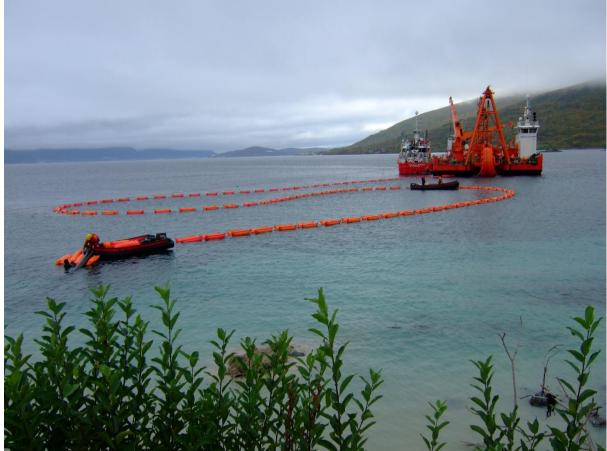
Figure 55 – Cable laying vessel shore landing installation
