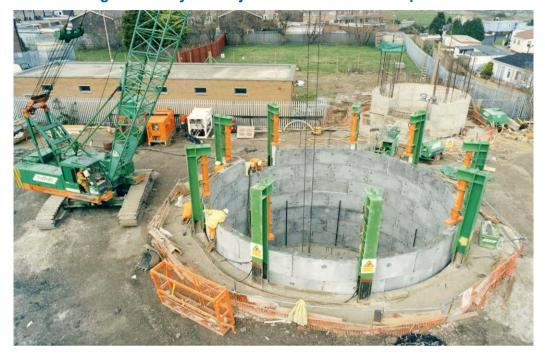
Figure 67 – Hydraulic jacks on caisson technique shaft construction
