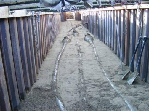
Figure 19 – EHV joint bay containing three Joints
