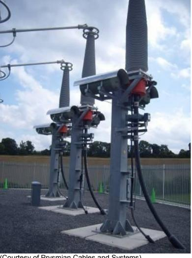
Figure 22 – 400kV terminations installed near Goring
