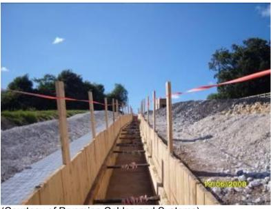
Figure 37 – A close-timbered cable trench
