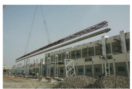
Figure 62 - GIL segment being lifted into position
