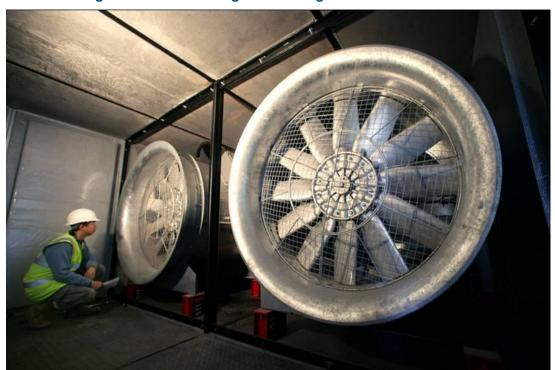
Figure 46 – Air cooling fans during installation
