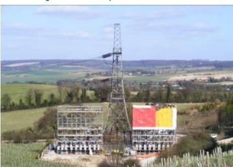
Figure 23 – Weatherproof enclosure for cable termination assembly
