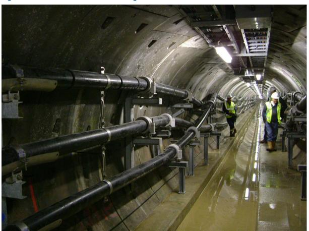
Figure 3 – 400kV cable tunnel crossing beneath the Thames at Dartford
