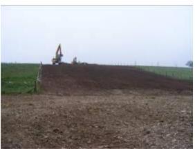
Figure 44 – Topsoil replacement
