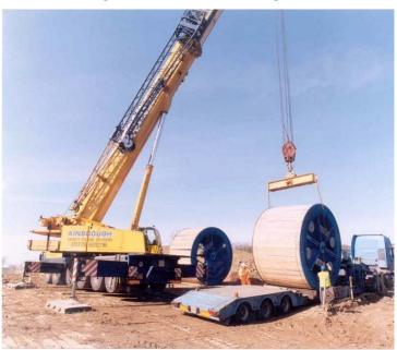
Figure 40 - Offloading cable drums
