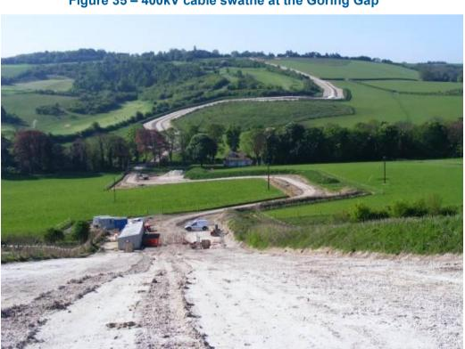
Figure 35 – 400kV cable swathe at the Goring Gap
